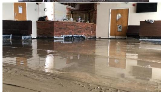
Part of the solution to fix the floor was to lay a screed of concrete to ensure it is even across the room before the oak laminate is laid. This work will hopefully be completed within the next couple of weeks.
